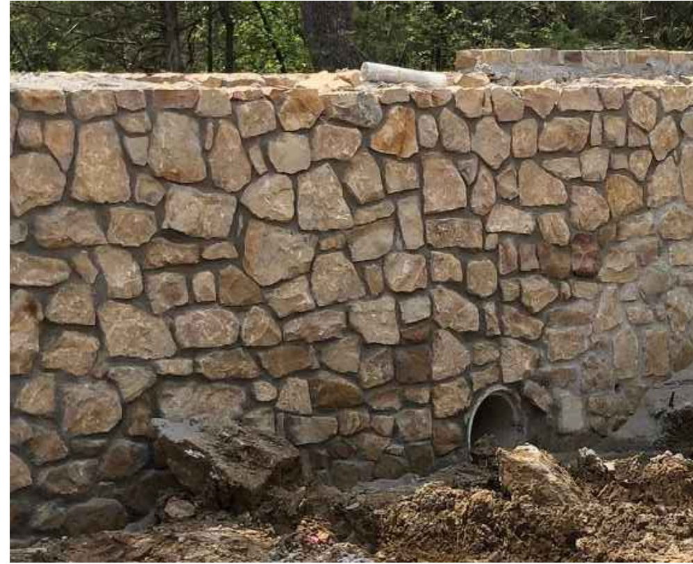
LAKESIDE CROSSING RETAINING WALL
