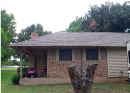
Transition from Brick to Hardi-Board around side and rear to match existing
