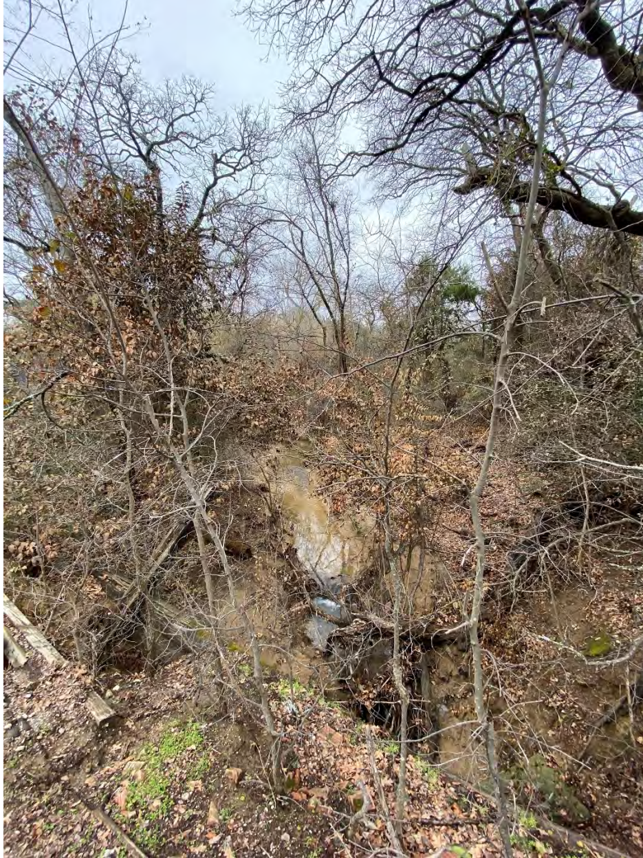
Creek running down middle of open space that electric and cable lines would need to run below.
