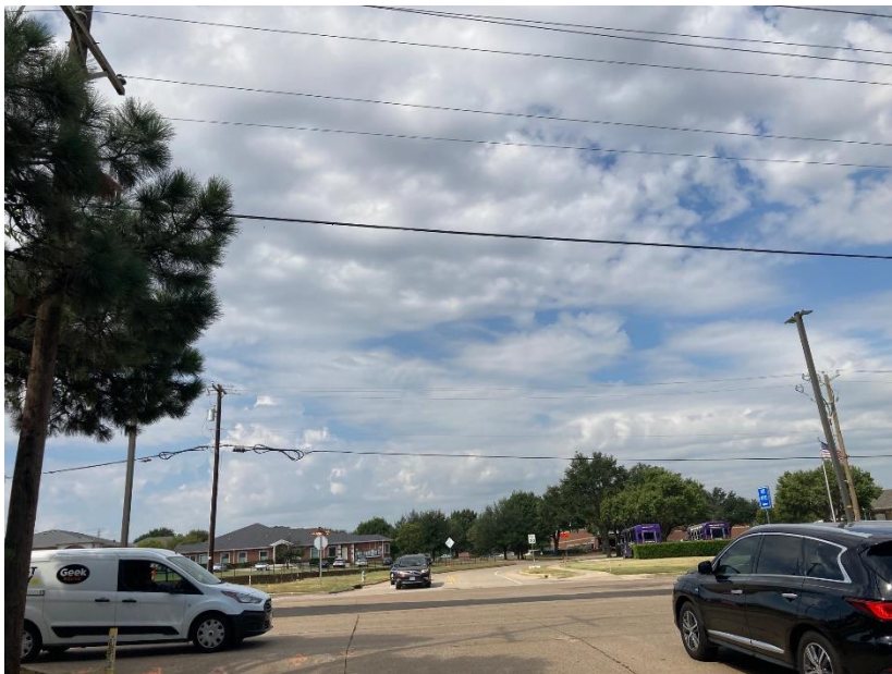
View from intersection with existing lines
