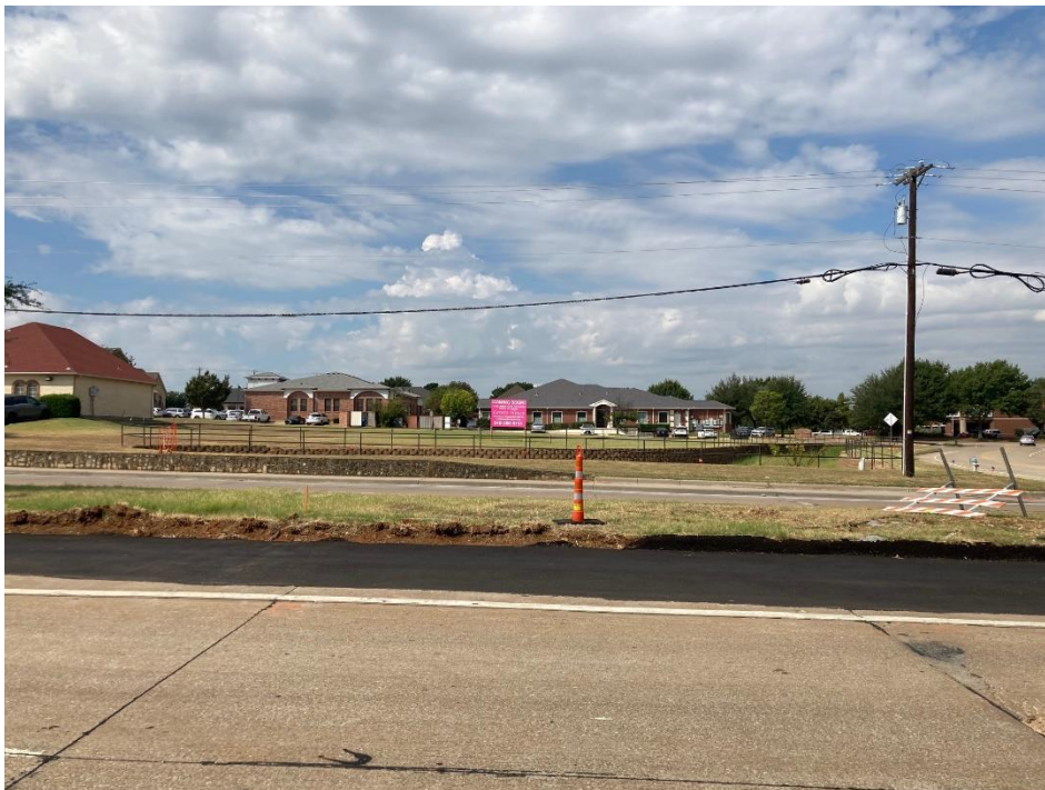
Morriss Street view with power lines.
