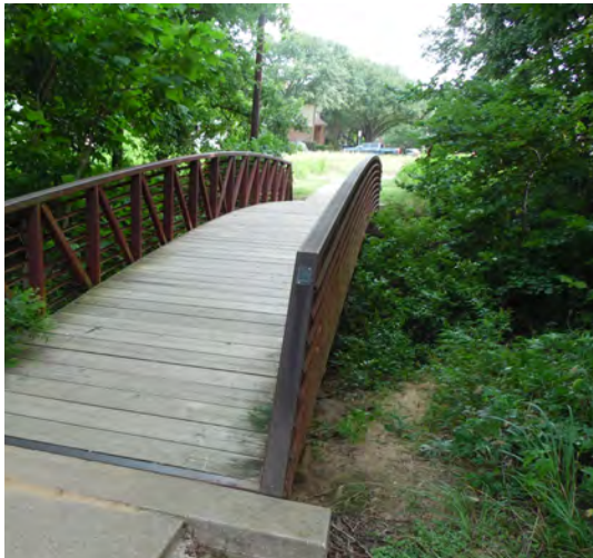
Pedestrian bridge over creek
