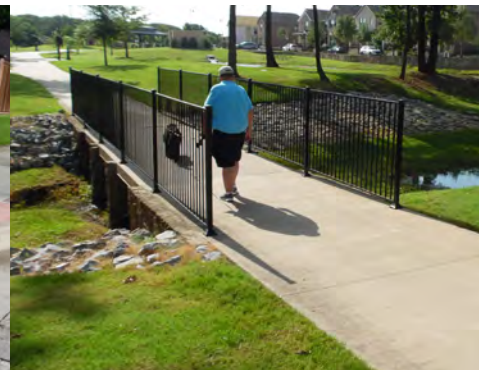
Trail bridge near Riverside
