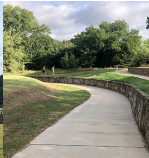
Retaining wall adjacent to trail
