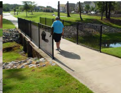
Trail bridge near Riverside
