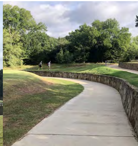
Retaining wall adjacent to trail
