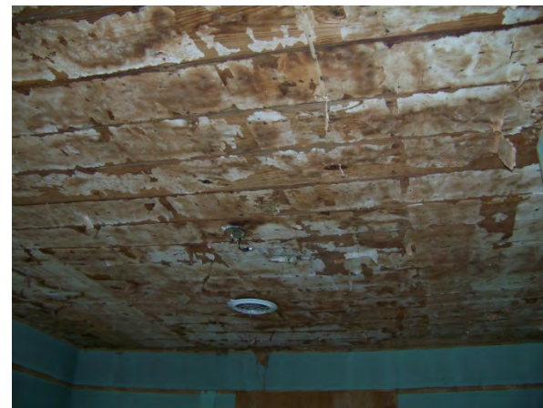
Interior view of ceiling wood planks and historic wallpaper
