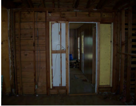
Interior view of the Kitchen looking north
