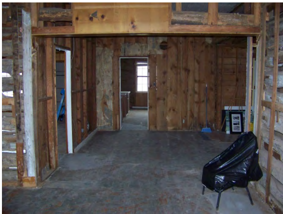
Interior view of south wall where historic entry would have been located
