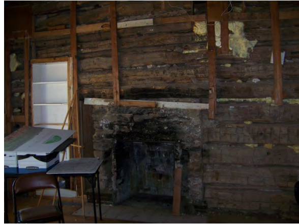
Log house visible from interior of house. Constructed between 1860 and 1861 is one pen measuring 16' x 16'.
