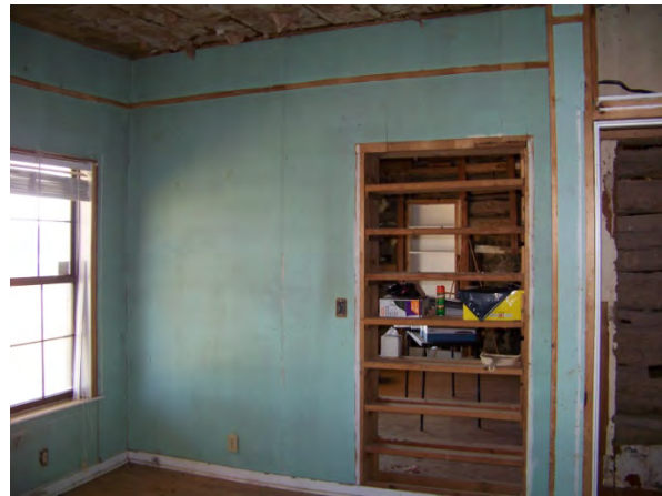
Interior view of east wall with opening to log house
