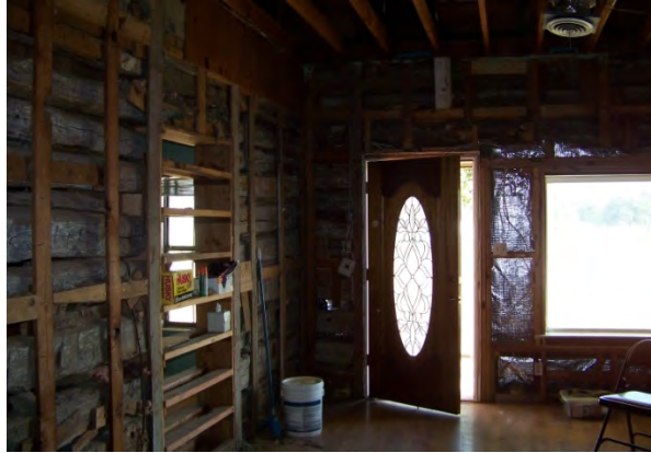
Interior view of west and north walls with current entry (north)
