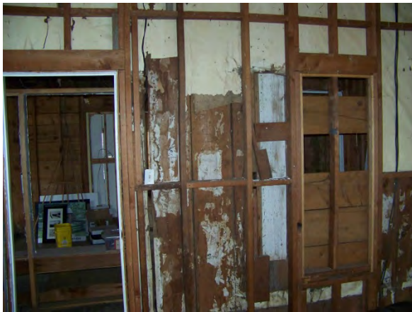
Interior view of south wall where historic entry would have been
