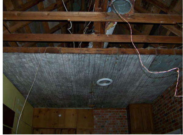
Interior view of the Kitchen ceiling looking north
