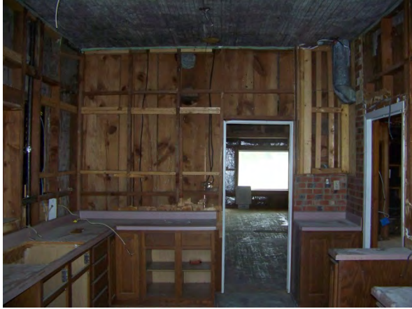
Interior view of the Kitchen looking north
