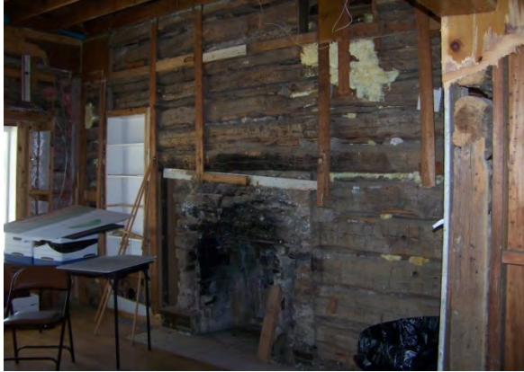
Interior view of east wall of the log house
