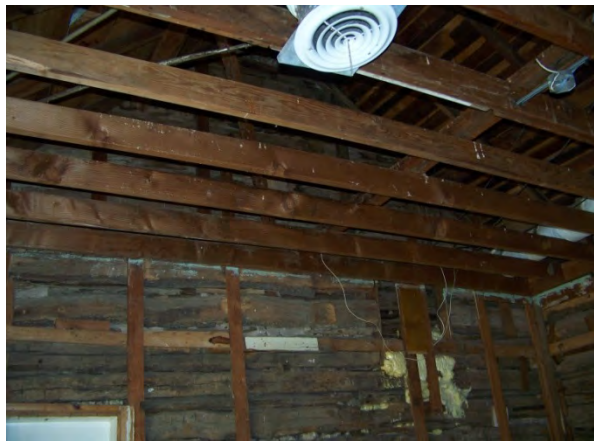
Interior view of newer ceiling structure and east wall
