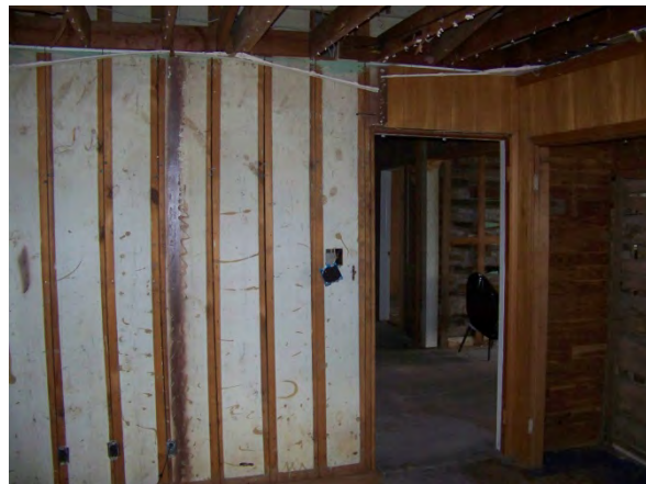
The third pen was constructed in clad with board and batten siding. The earlier two pens remained clad with clapboard siding.
