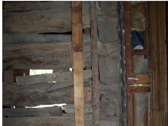
When the second pen was added to the west of the log house, the entire house was clad in clapboard siding. This siding can be found within the east and west walls of the house.
