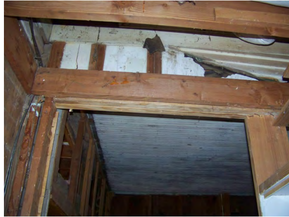
Small additions to the house occurred prior to the addition of the tear-drop siding. Photograph above shows the tear-drop siding cut at the angle of one of the roofs and remnants of asphalt shingles.
