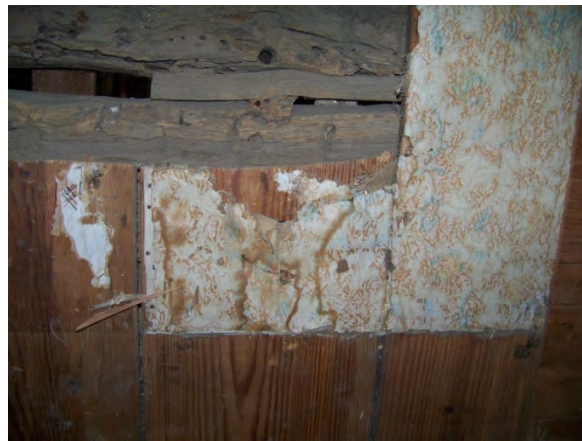
Interior view of closet wall with historic wood planks and historic wallpaper, with cut-out to log house wall
