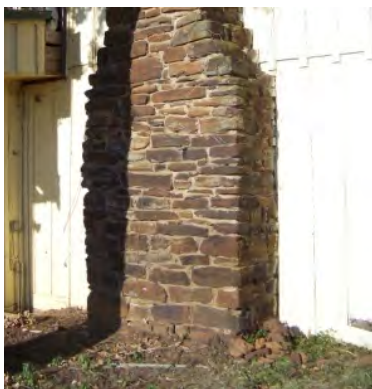
Existing chimney built of red sandstone, presumably quarried locally
