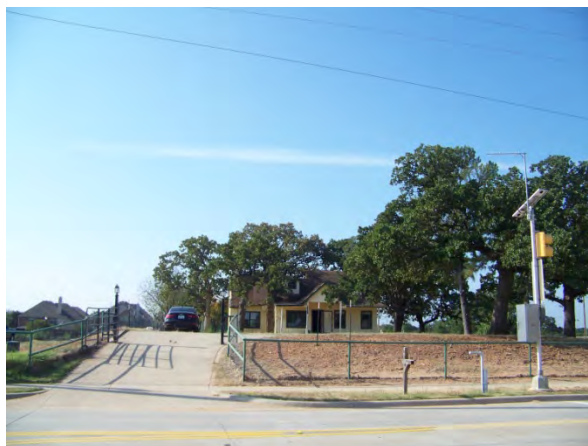
Fence and gate at Quail Run
