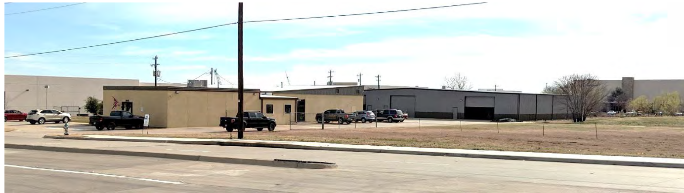
West Elevation – Building 1 / North & West Elevation – Building 2
