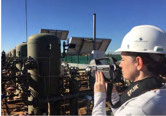
Near-Equipment Inspection efforts during a padsite inspection event using an Optical Gas Imaging (OGI) Camera to record a leak.
