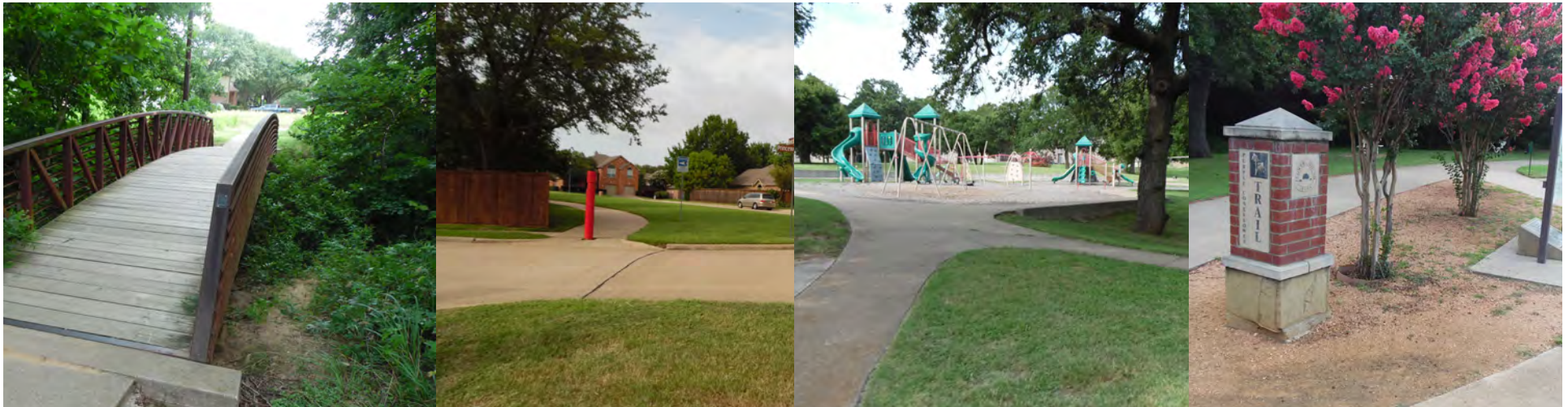
Pedestrian bridge over creek
