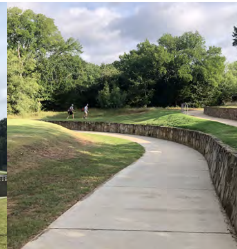
Retaining wall adjacent to trail
