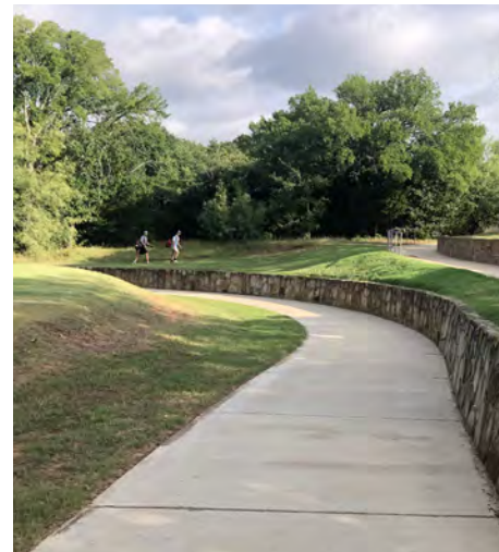
Retaining wall adjacent to trail
