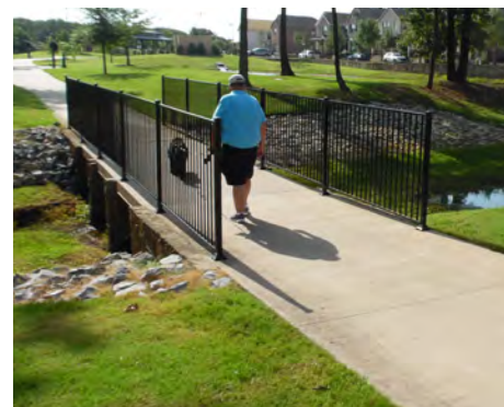
Trail bridge near Riverside
