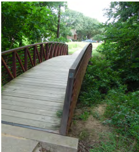
Pedestrian bridge over creek
