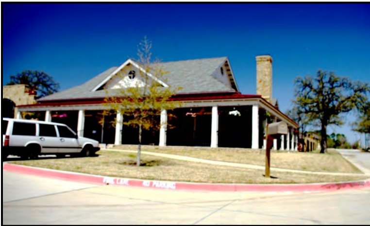
Examples of Compliant Pitch Roof:
