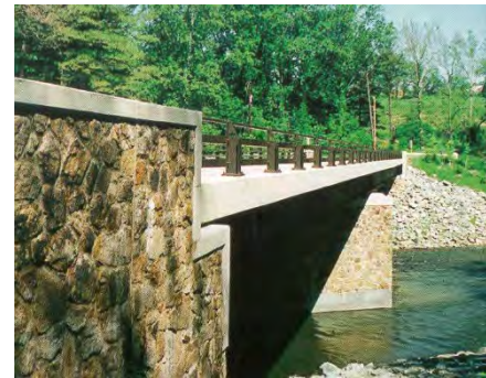
District arterial bridge enhancement
