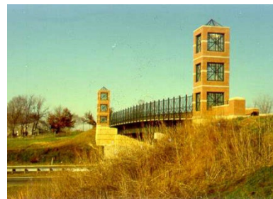
Enhanced arterial bridge treatment with sidewalk example
