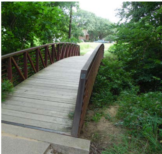
Pedestrian bridge over creek
