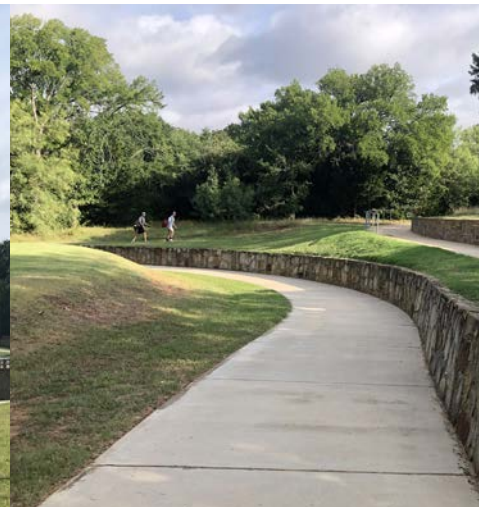
Retaining wall adjacent to trail
