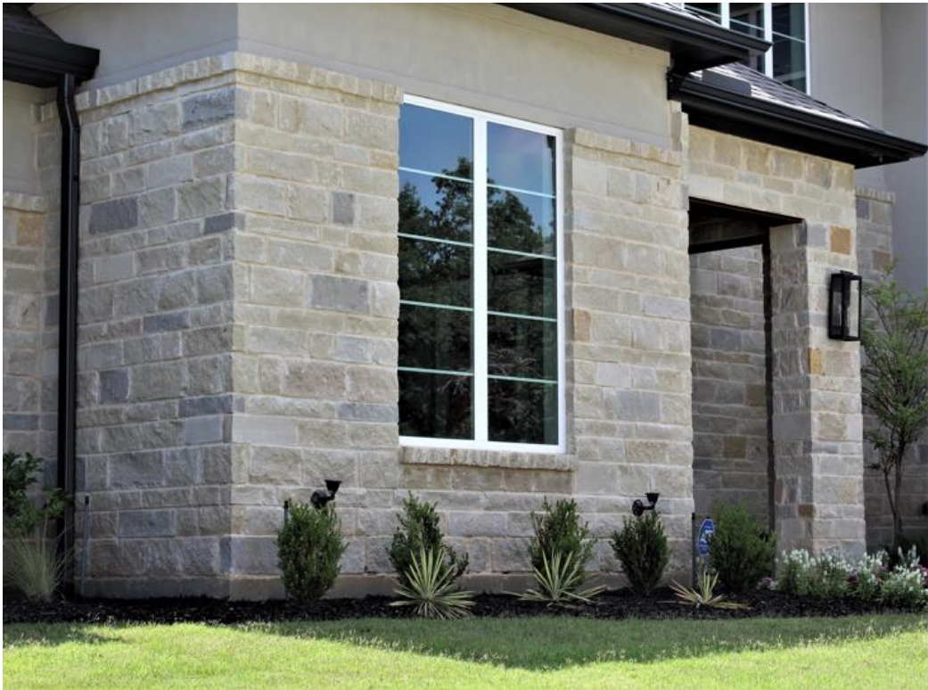
Buff Smoke Blend Installed
