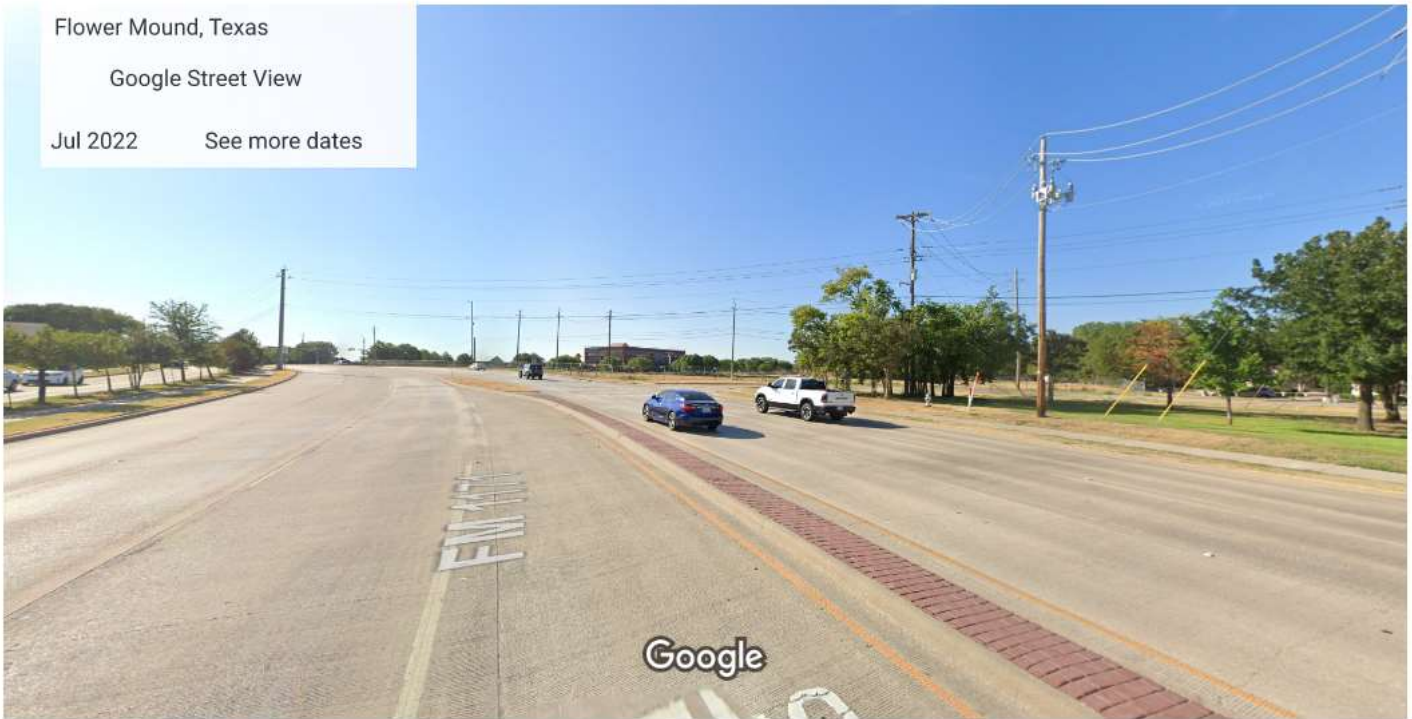
3100 FM 1171 with power lines
