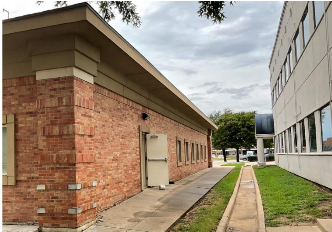
NORTH EXISTING EXTERIOR
