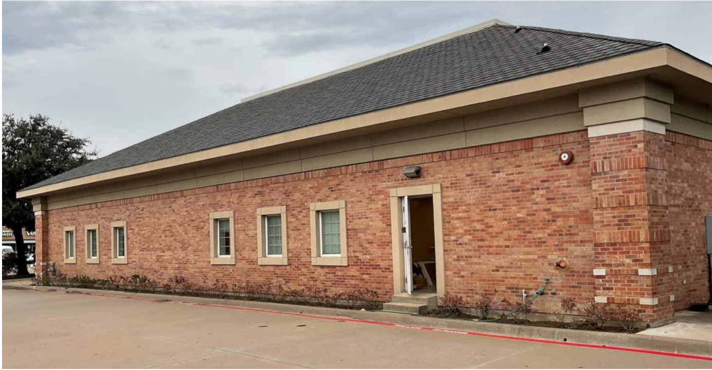
SOUTH EXISTING EXTERIOR
