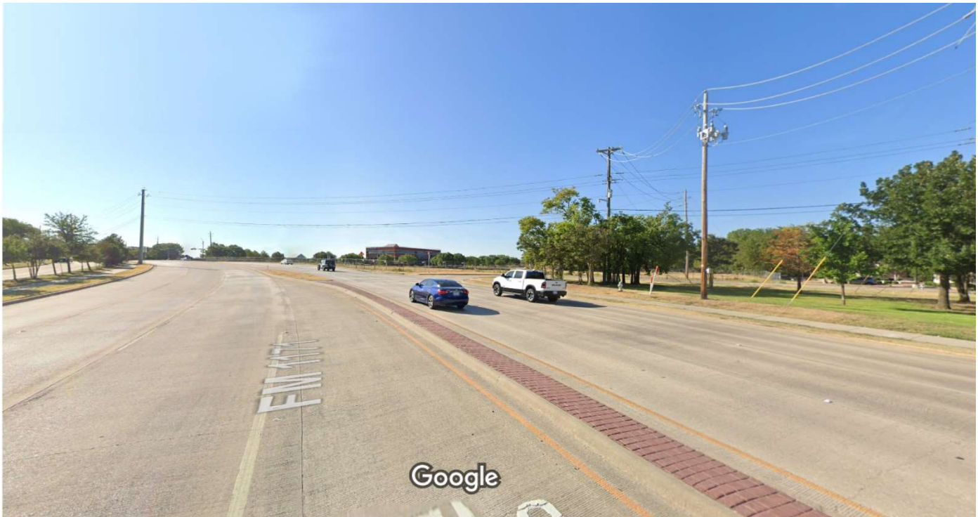
3100 FM 1171 view without power lines
