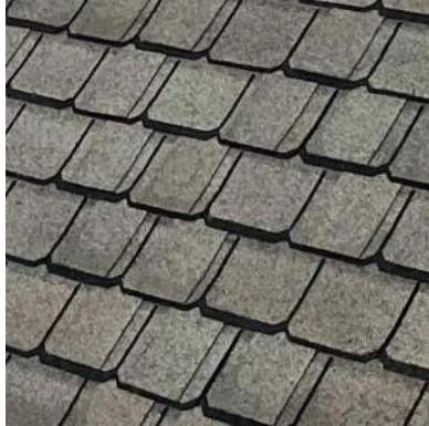
EXISTING GRAY SHINGLE ROOF
