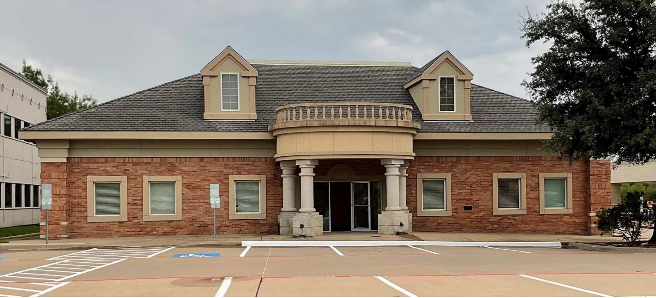
WEST EXISTING EXTERIOR
