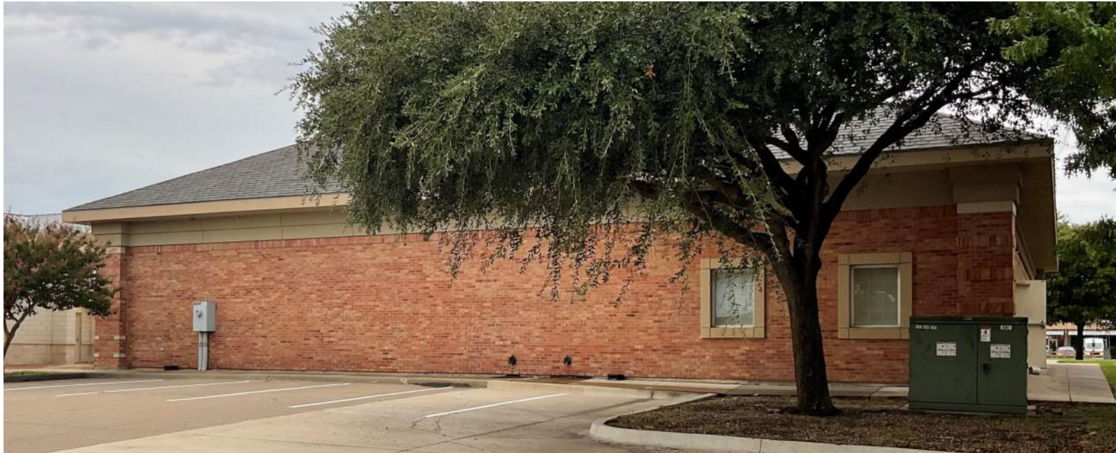
EAST EXISTING EXTERIOR
