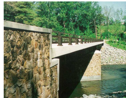
District arterial bridge enhancement
