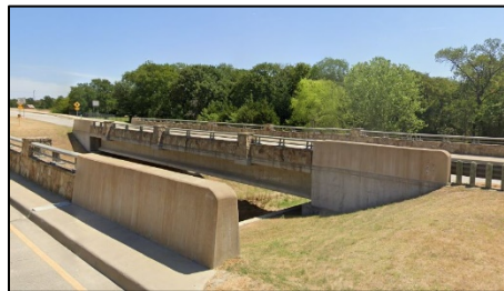
District-Minor arterial bridge enhancement
