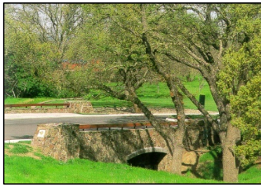
District Minor arterial bridge enhancement
