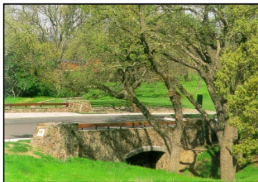
District-Minor arterial bridge enhancement
