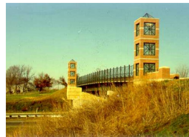
Enhanced arterial bridge treatment with sidewalk example
