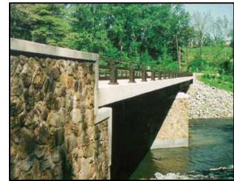
District Minor arterial bridge enhancement
