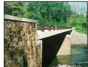
District-Minor arterial bridge enhancement
