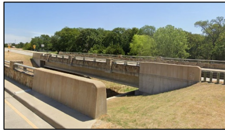
District Minor arterial bridge enhancement
