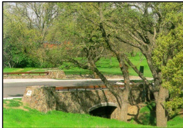
Minor arterial bridge enhancement
