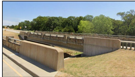
Minor arterial bridge enhancement
