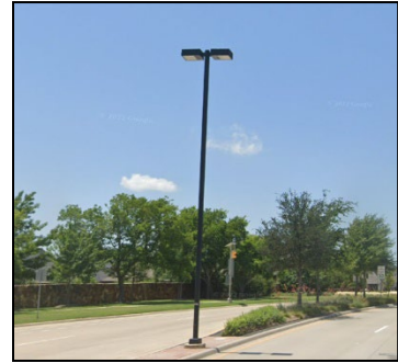
Example of existing light fixture light fixture
