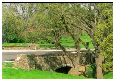
Minor arterial bridge enhancement
