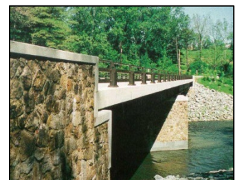
Minor arterial bridge enhancement
