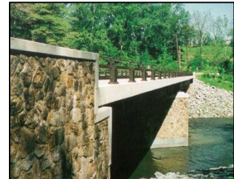
Minor arterial bridge enhancement
