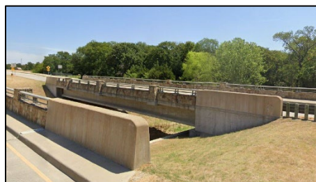
Minor arterial bridge enhancement
