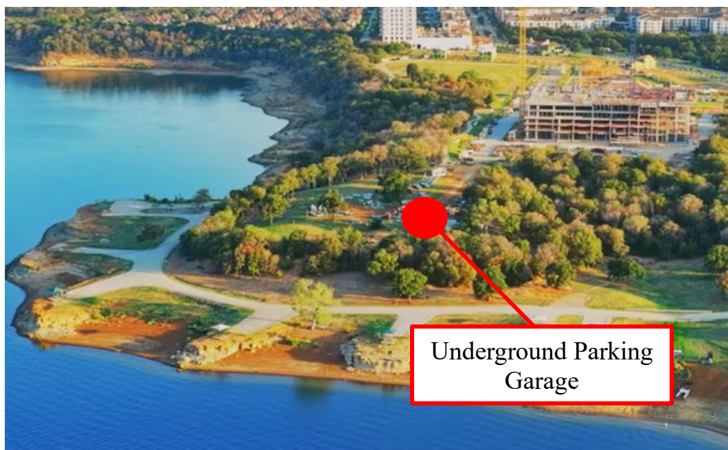
Figure 2: Drone footage of the parking garage site, facing north. The dense trees on the Corps' Lake Grapevine property screen the site from Rockledge Park in Grapevine. The red box outlines the approximate location of the garage.
