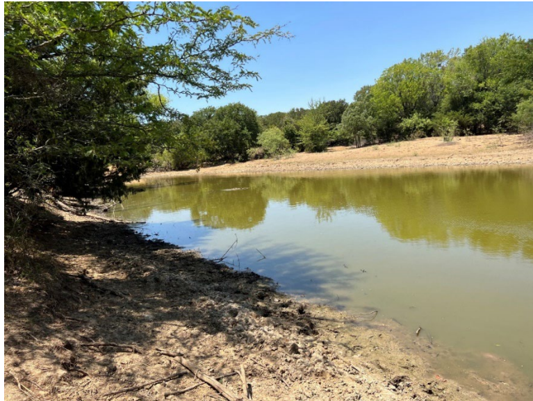
Pond 4 – an impoundment of the Unnamed Tributary to Denton Creek
