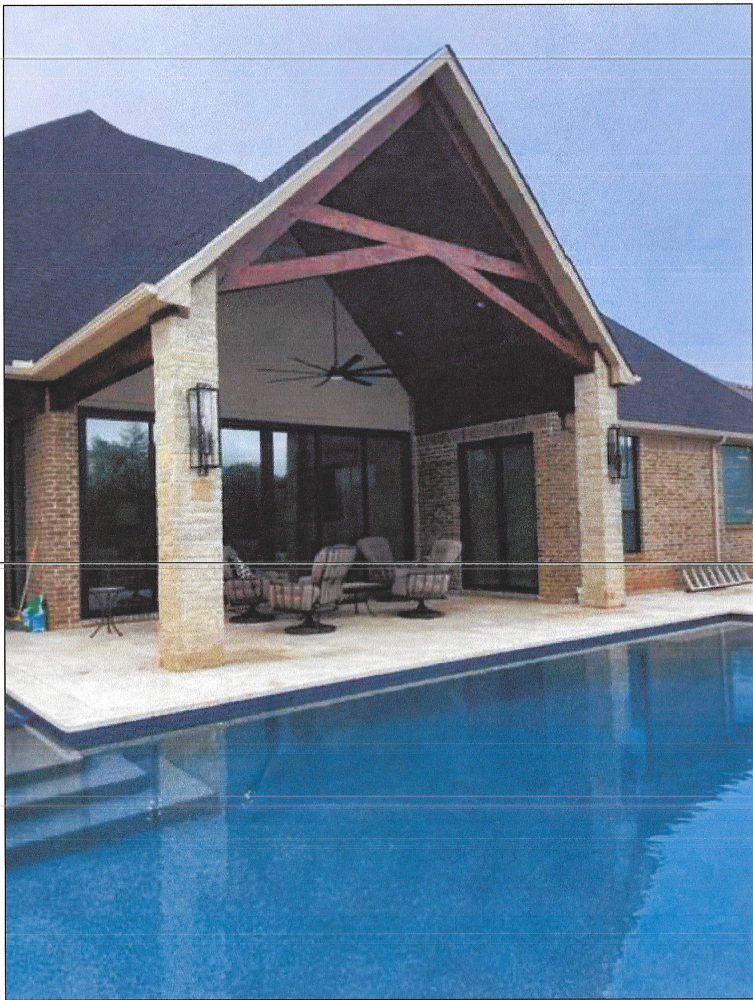
EXISTING VIEW OF REAR COVERED PORCH WITH WOOD BEAM DETAIL, STONE COLUMNS AND BRICK VANEER.
