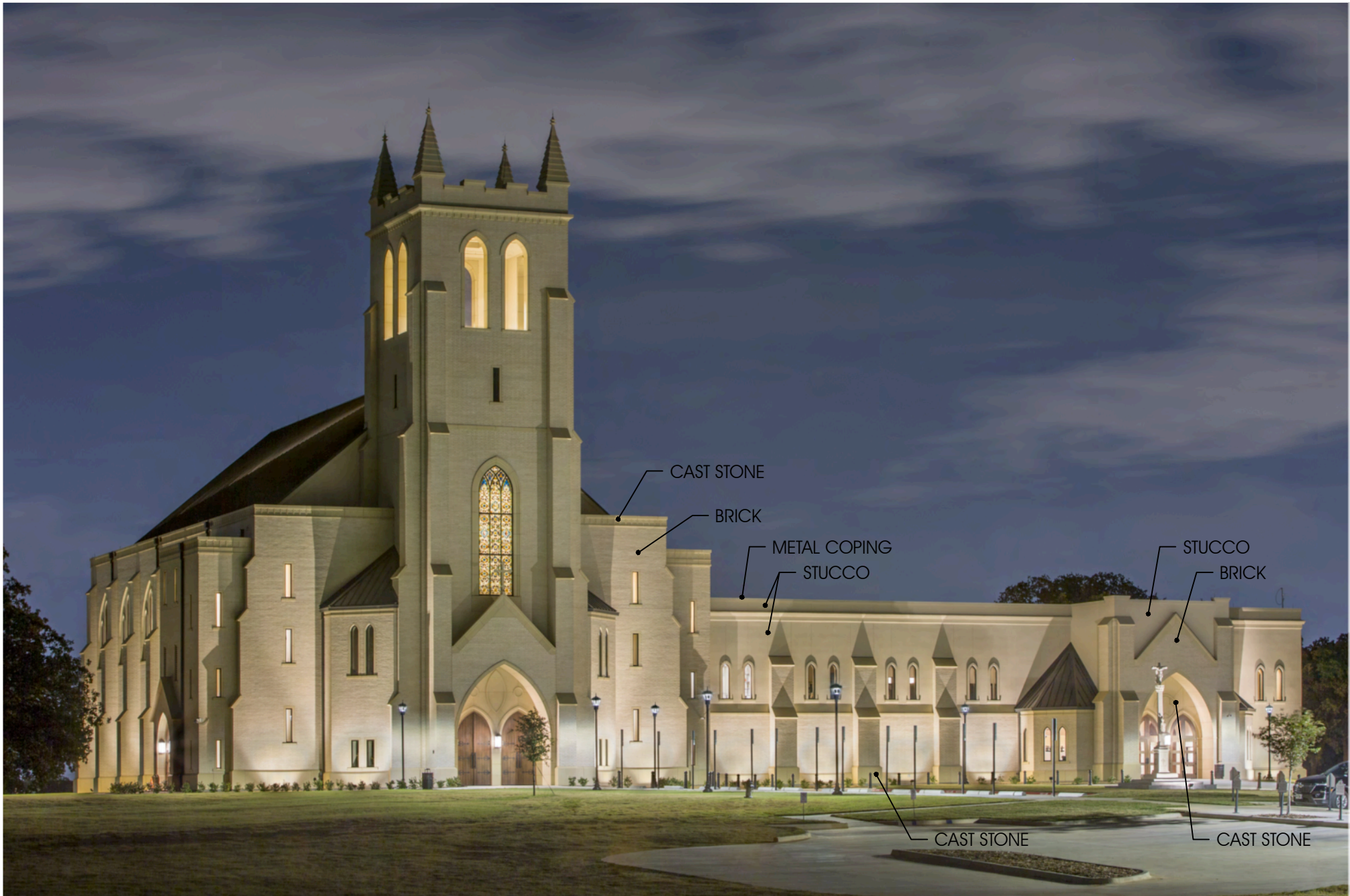
2 PHOTO - EXISTING CHURCH EXTERIOR MATERIALS - WEST ELEVATION
