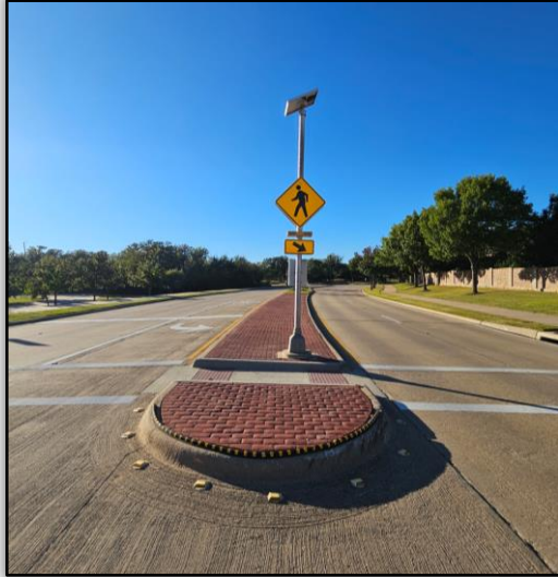
Figure 9. Pedestrian Refuge Island at a Marked Crosswalk Source: Town of Flower Mound, Tx
