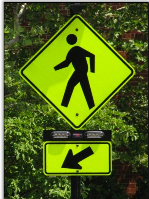
Figure 11. Close-up View of an RRFB
