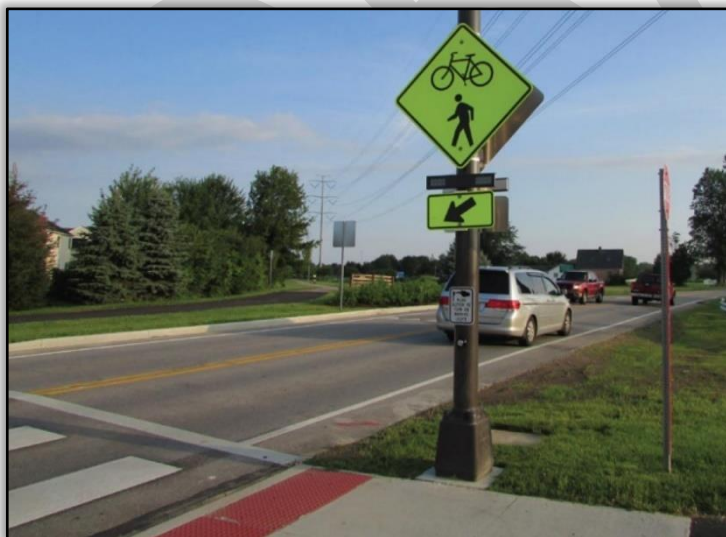
Figure 10. RRFB Installed at a Marked Crosswalk (Approach View)
