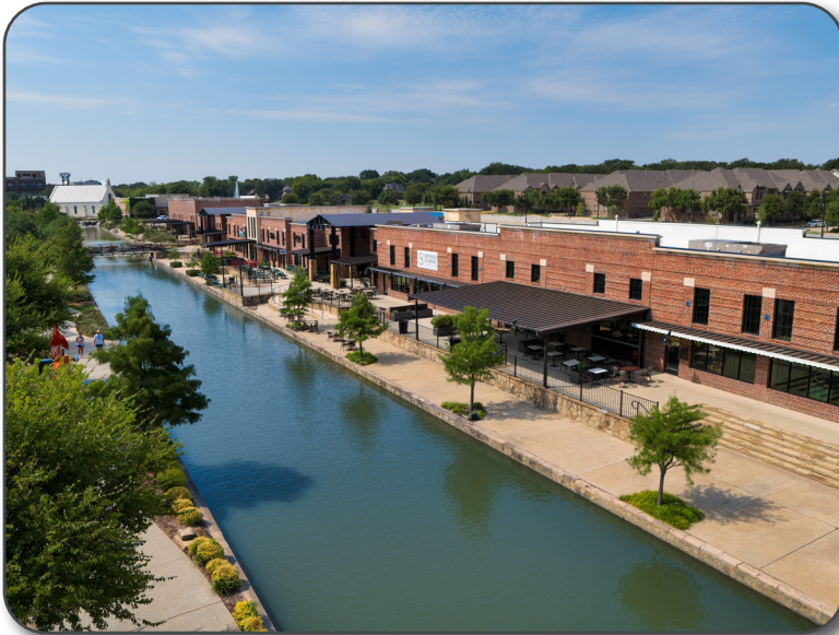
A view of the River Walk's Restaurant Row containing 23,570 square feet of restaurant space. The development includes a mix of uses such as retail, office, residential, hotels, and event spaces.
