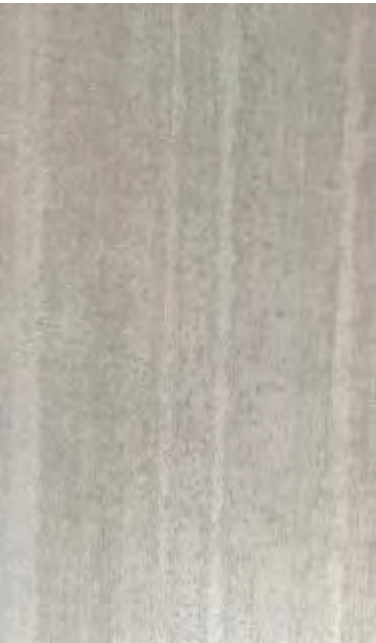
Paint-1 Painted/Textured Concrete
