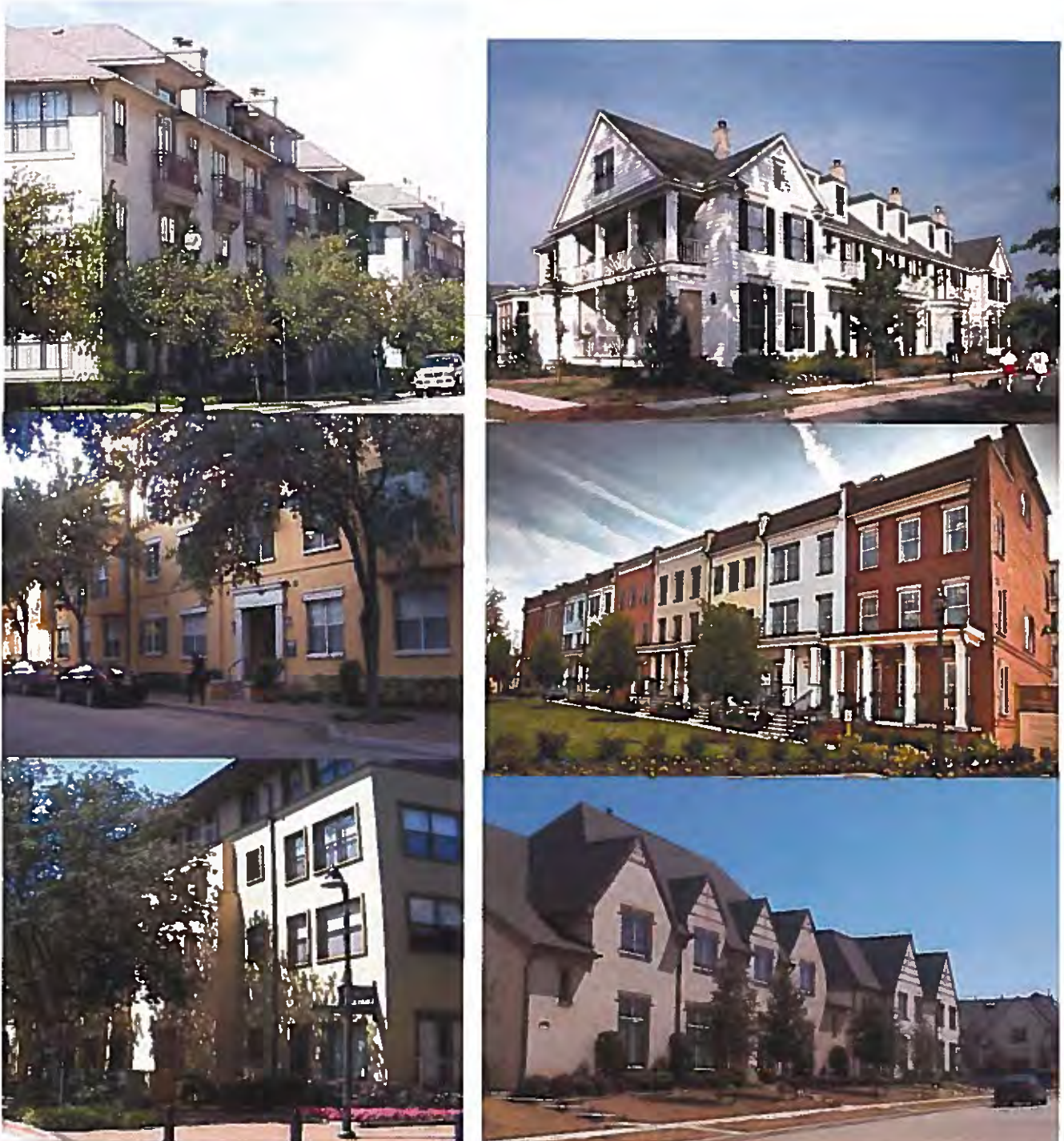
Figure 7.5: Residential Multifamily and Townhome Structures
