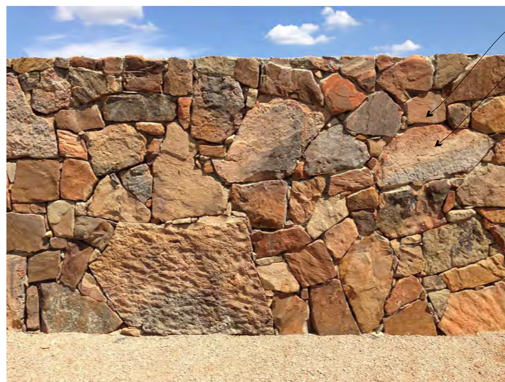
TYPICAL WALL STONE & JOINT SIZE, SHAPE, TYPE & PATTERN
